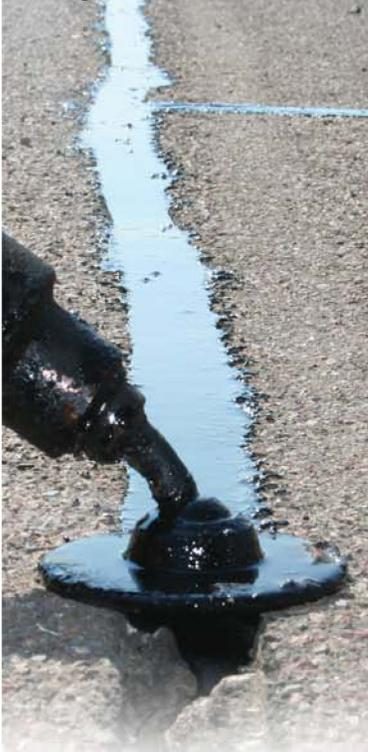
**P**avement is a costly investment. Just as you would seal leaks in the roof of your building, you should seal cracks in your pavement. Water infiltration through cracks causes deterioration of the pavement and substructure. Untreated cracks propagate and multiply, developing potholes. The result is expensive repairs and reconstruction.
