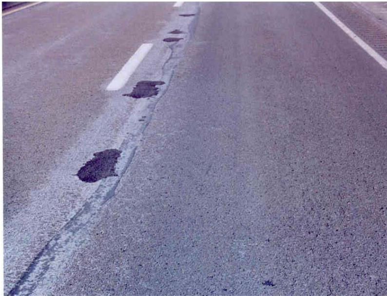
Figure 1. Deteriorating Longitudinal Joint
