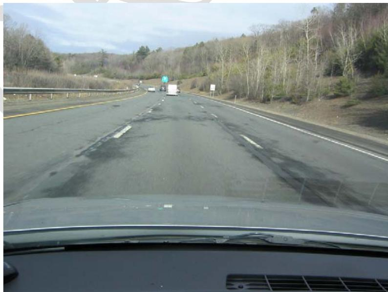
Figure 2. Longitudinal Joints That Are Permeable and Failing
